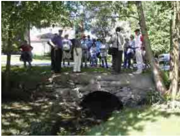
Zone 2 – Undersized Culvert
